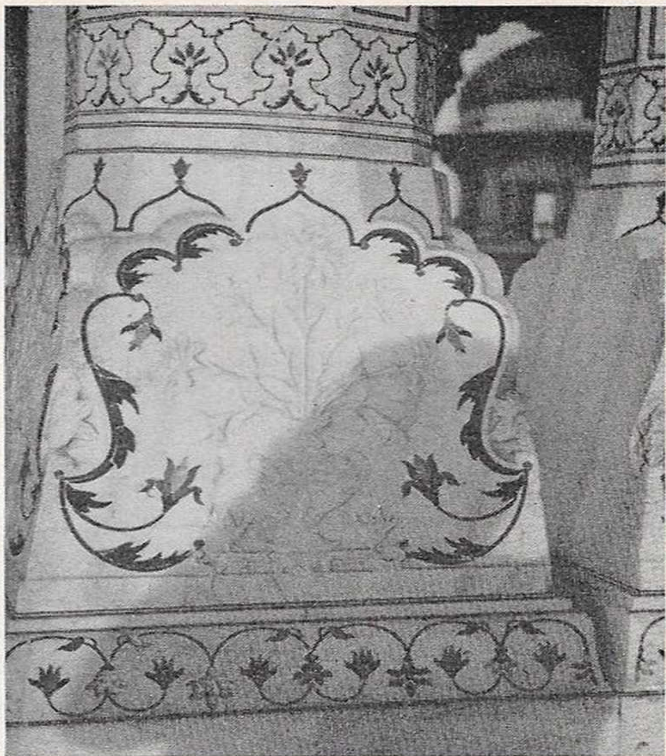
Carved pillar in Agra Fort, inlaid with red, green, and blue stones. Tourists have taken as souvenirs all the colored inlays from the center of the design.
